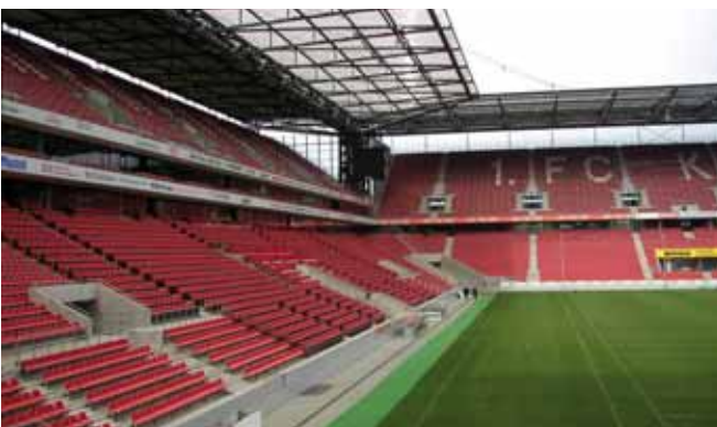
Fixing of safety rails, Rheinenergiestadion Cologne
