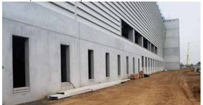
UPS Air Hub, Cologne Bonn Airport, Germany
