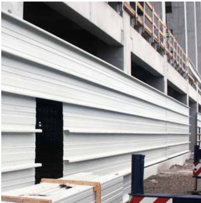
Façade fixed using HALFEN HTU Cast-in channels
