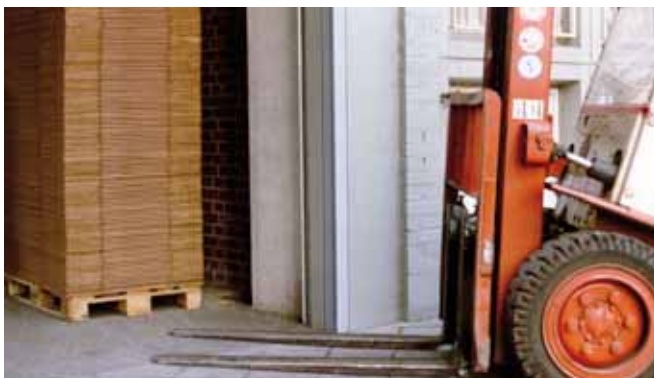
Corner guards in an industrial environment
